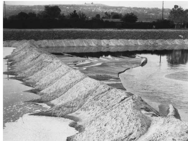
Reconstructed sand levee in the river
