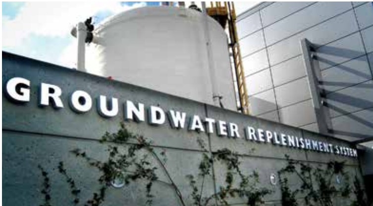
Groundwater Replenishment System building
