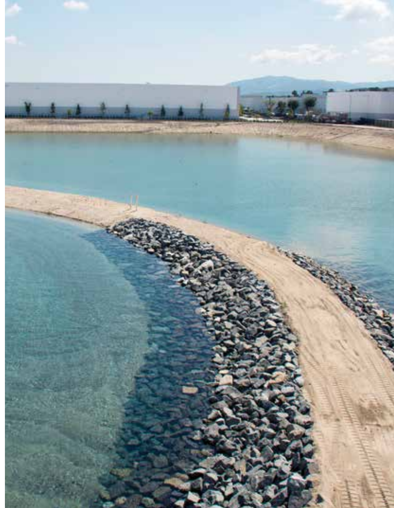
La Palma Recharge Basin in Anaheim
