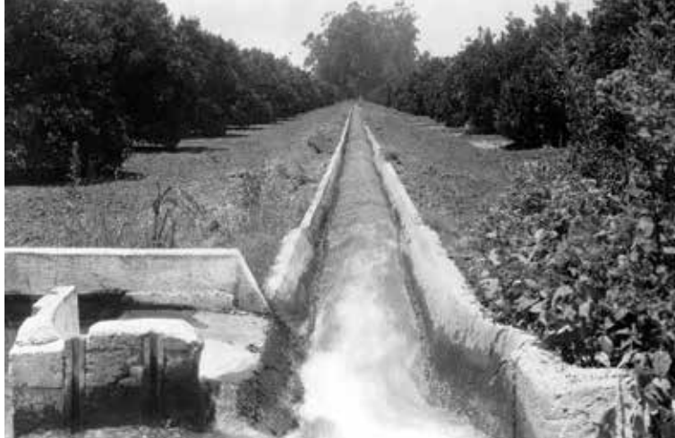
Open canal of the Anaheim Union Water Company, photo courtesy of Santa Ana Public Library
