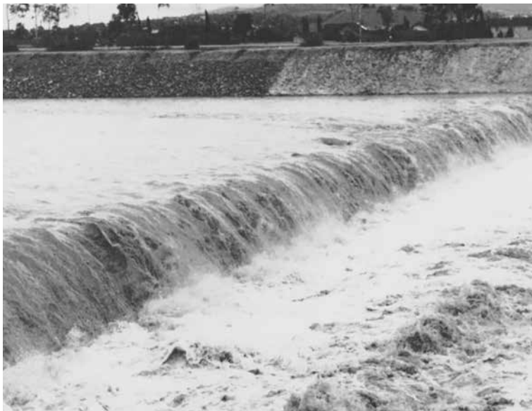
Storm flow spilling over a drop structure en route to ocean
