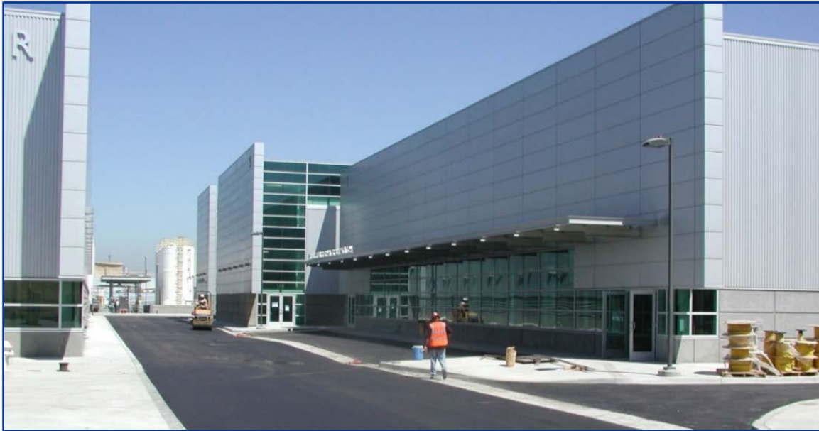
Figure 2-25. Barrier and Product Water Pump Stations
