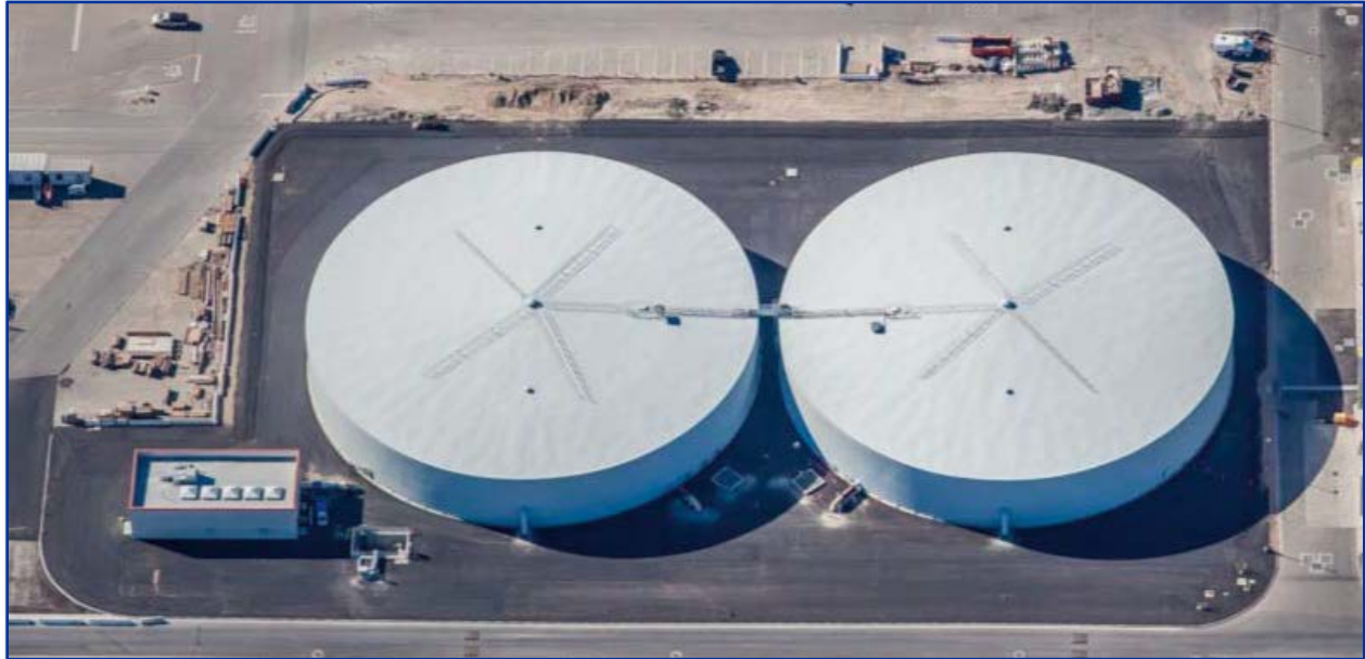
Figure 2-3. OC San Plant 1 Secondary Effluent Flow Equalization (SEFE) Tanks and Pump Station
