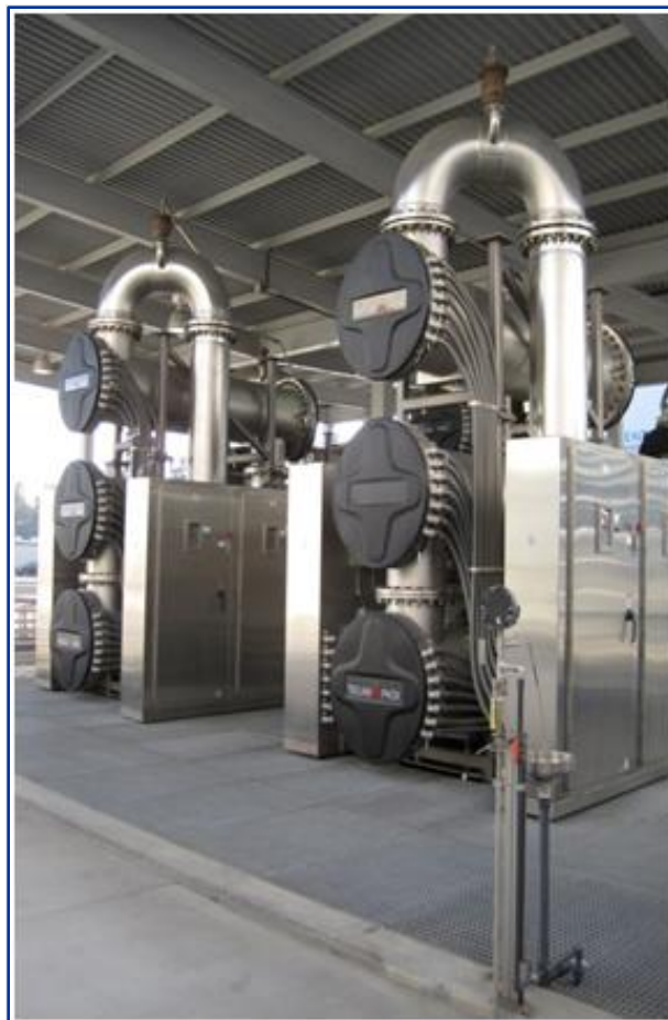
Figure 2-20. UV/AOP System
