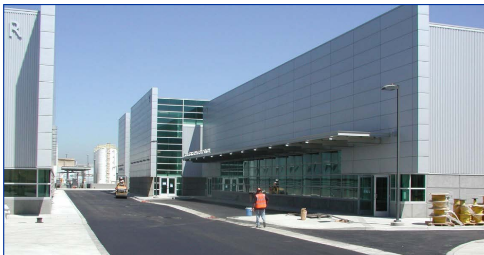
Figure 2-17. Barrier and Product Water Pump Stations
