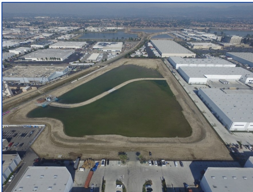
Figure 5-3. La Palma Basin with GWRS Purified Recycled Water in 2016
