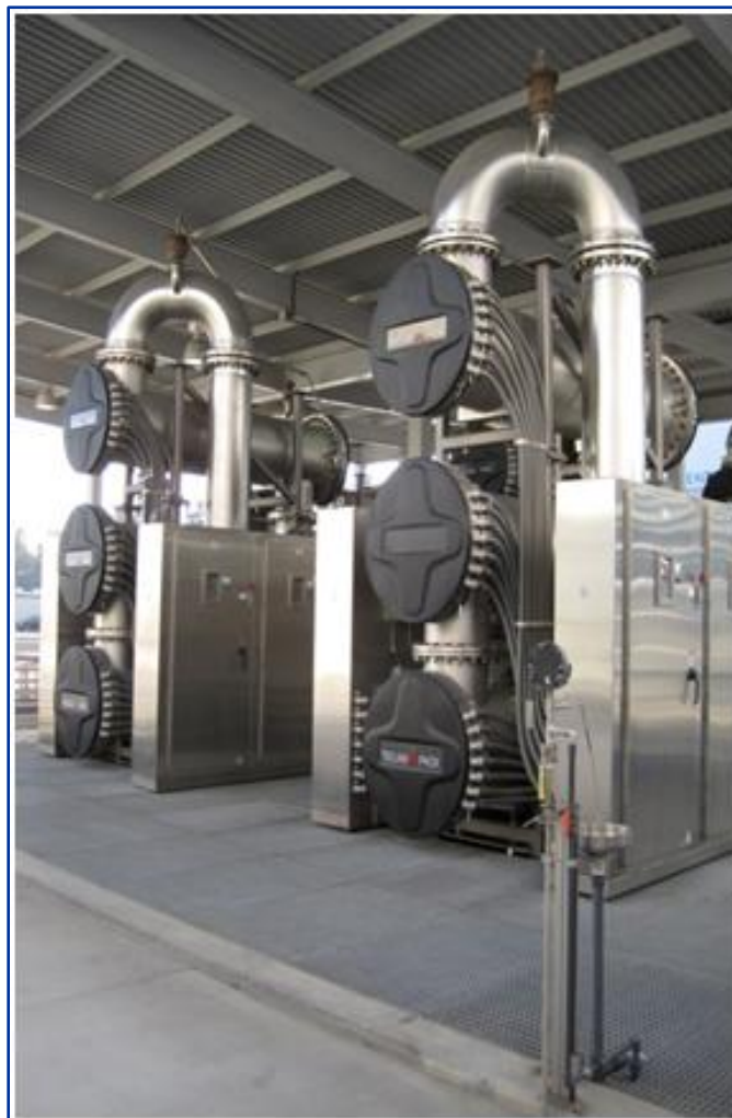
Figure 2-12. UV/AOP System
