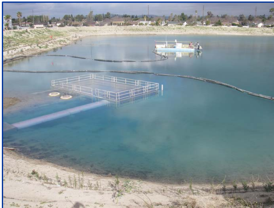
Figure 5-1. Miller Basin with GWRS Purified Recycled Water in 2008
