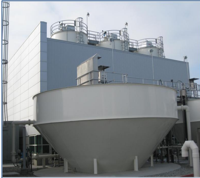
Figure 1-10. Lime Post-Treatment System
