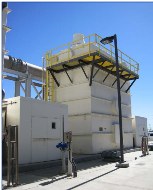
Figure 1-9. Decarbonation System
