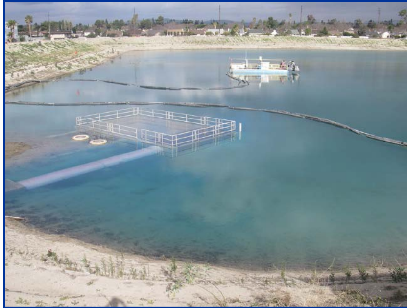
Figure 1-17. Miller Basin with GWRS Purified Recycled Water in 2008
