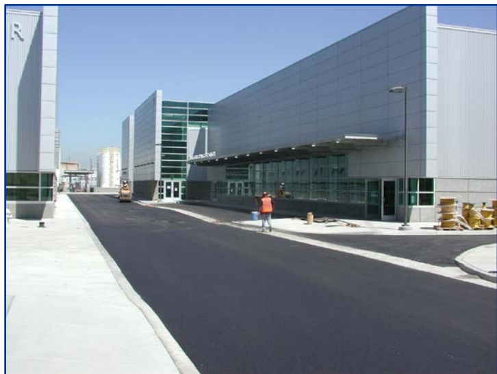
Figure 1-11. Barrier and Product Water Pump Stations
