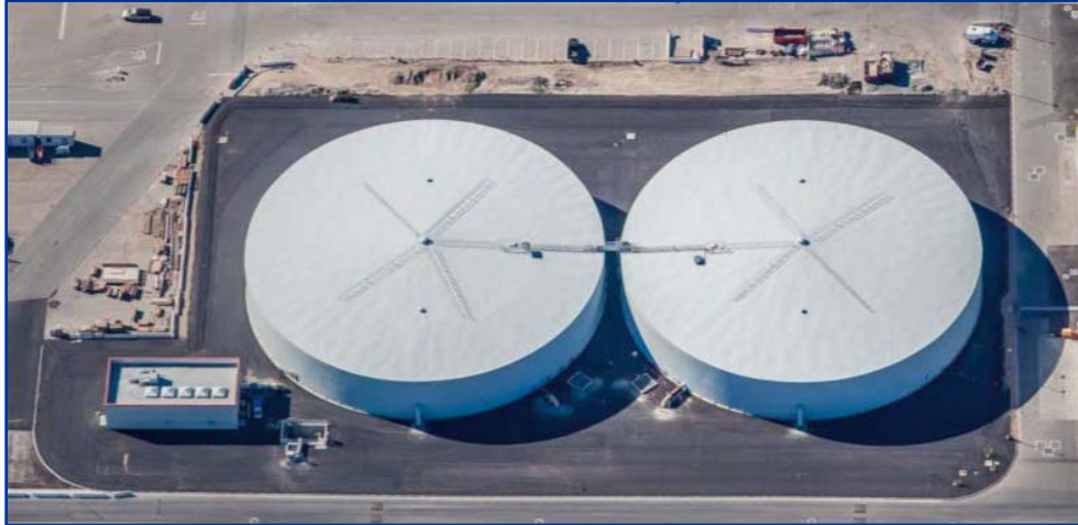
Figure 1-5. Secondary Effluent Flow Equalization (SEFE) Tanks and Pump Station
