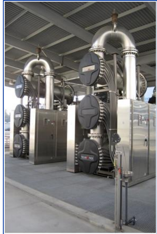
Figure 1-8. UV/AOP System
